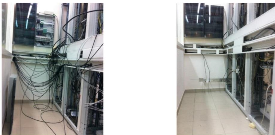
View of the ROB Time Laboratory in January 2017 (left) and December 2017 (right); a surge protection system was installed in 2017 through the metallic plate visible on the lower part of the wall in the picture on the right hand side
